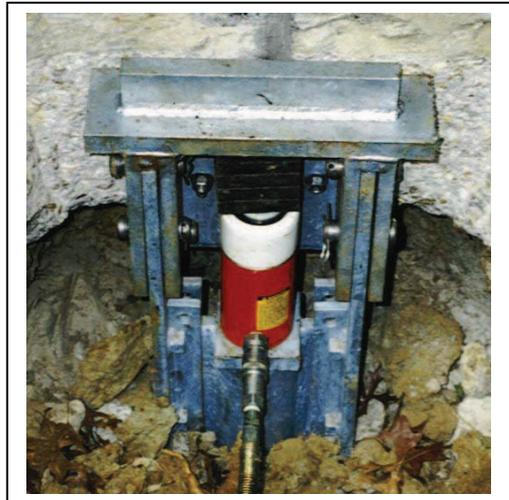
When all piers have been installed, the manifolds and hydraulics are loaded uniformly as much as possible (see photo at bottom right). Upon transfer of load to the entire pier assembly, lift pressures are
