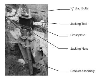
12. Place the jack or hydraulic cylinder between the T-Pipe and the cross-plate on the jacking tool. Adjust the height of the jacking tool as required to meet the height of the jack.
