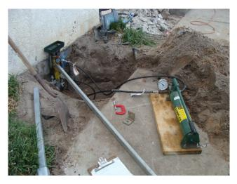
13. Apply a small amount of pressure to the jack, just enough to take up the "slack" in the assembly. Once again, check to see if the bracket is still mounted flush with the foundation. Tighten the cross-bolt if necessary and check the bracket mounting bolts again before proceeding.
