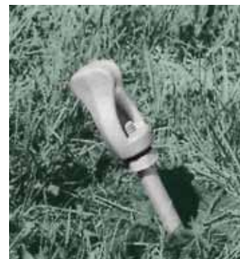
Install eye nut and secure guy.
