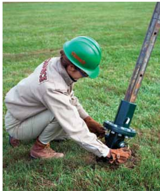
With anchor at proper depth, release tooling.
