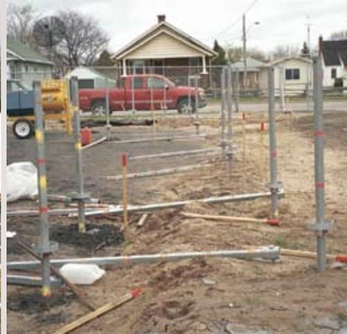
Helical lead sections have been installed. Extensions with a Lead Displacement Plate are ready for installation with grout reservoir.
