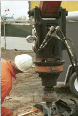
Monitoring torque during installation confirms bearing capacity.
