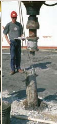
Pulling out the grout reservoir after reaching the specified torque.
