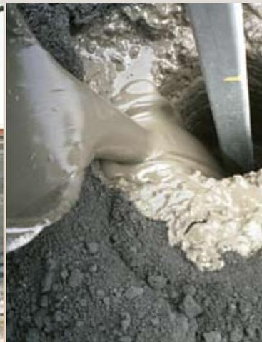
A Helical Pulldown® Micropile is a displacement pile that forces the soil out around the shaft. The void is filled with grout.
