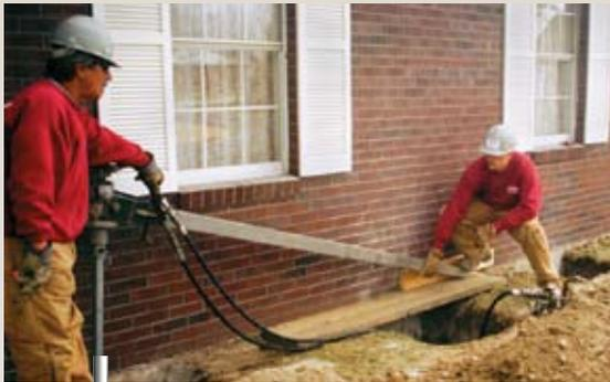
Installation of the micropile is completed quickly and easily with a hydraulic torque motor mounted on readily available equipment. Challenging sites, even with limited access, are overcome with the Helical Pulldown® Micropile.
