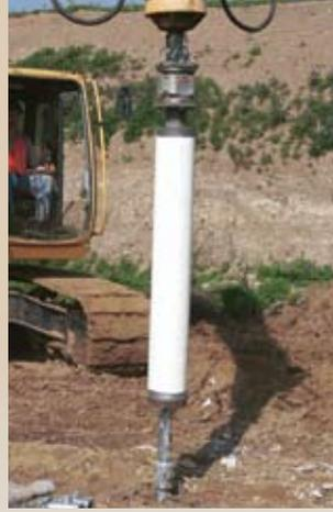
Installing an extension with Lead Displacement Plate and PVC grout reservoir.
