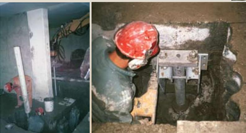
Adding an extension to get to founding depth and installing a repair bracket. The PVC casing minimizes negative down-drag forces.
