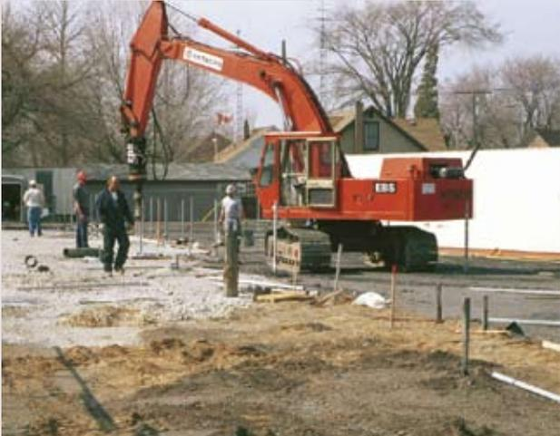
An excavator with torque motor installs a row of Helical Pulldown® Micropiles to support a new building.
